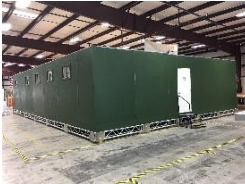
Figure 4: RDS for US government contract, configured for office, barrack, and recreation
