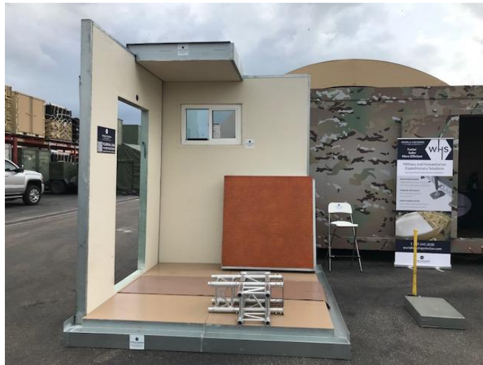
Figure 1: Cut-away view of Rapidly Deployable Structure (RDS) comprised of insulated Rapidly Deployable Insulated Panels (RDP) as demonstrated by World Housing Solution at SOFIC
