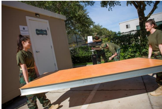
Figure 2: Lightweight RDP panels are used for all structural elements.
